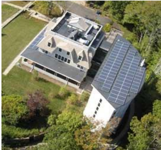
Aerial view of the Ordway Building, showing 2-part array of 88 photovoltaic panels. Photo courtesy Charles C. Benton.
