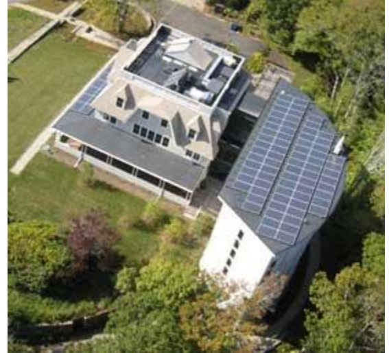
The Woods Hole Research Center's high-performance building with roof-mounted photovoltaic panels (photo credit - Chris Benton).
