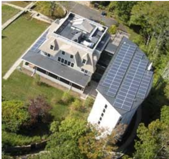
Aerial view of the Ordway Building, showing 2-part array of 88 photovoltaic panels. Photo courtesy Charles C. Benton. Select image for large version (154KB).
