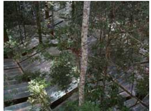
Overhead view of the panels
